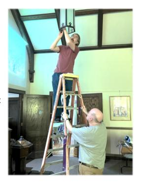
Now, 11 years later, we replaced the eight CFL bulbs with LED bulbs which Jim Shatek obtained at Lowes. They cost less than we originally paid for the CFLs, (and less than the original incandescents) and use just 36 Watts apiece, for a total of 288 Watts. Also, these bulbs have a life span of 15,000 hours compared to a life span of only 1000 hours for the original incandescent bulbs. We've come a long way from 2.4KW!
